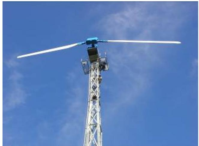
The standard total height of the tower is 30 metres (as an option a 40-meter tower is also available). The tower has an external ascent, and is provided with a steel cable parallel to the ladder in order to connect the fall-protection gear of the maintenance engineer as a safety measure. The tower is made of hot dip galvanised steel.
